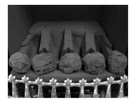
d) Select four of the large coals and arrange behind the front row of coals, ensuring that flame paths as indicated below are not interrupted. (See fig. 4 below)
